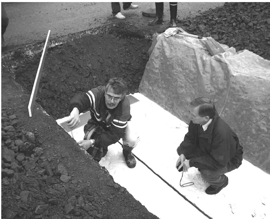
Figures 3b. Exposed EPS-surface in the test pit on Pesurinkatu.
